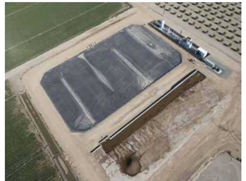
An Aerial View of an Anaerobic Digester
