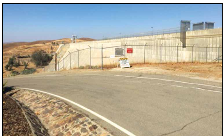
Friant Dam is triangle shaped and about a mile long at the top.
